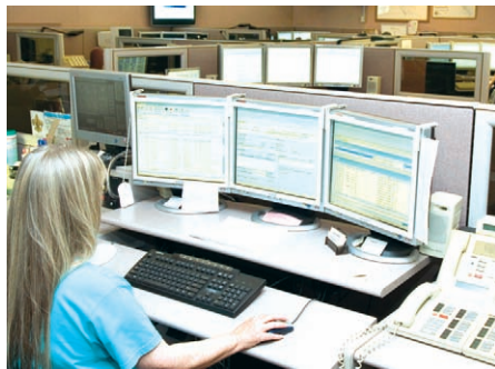
LCWC supervisor position where shift supervisors use Forge CAD to easily observe and oversee any active or completed incident details.
